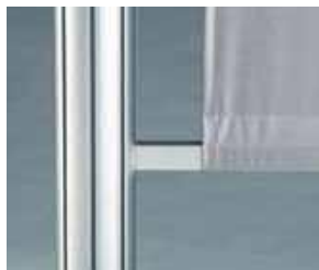
Connection of upright and beam
